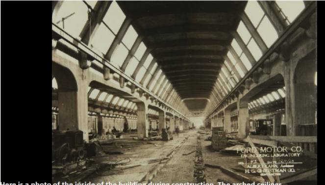
Here is a photo of the inside of the building during construction. The arched ceilings contained over 65,000 sq. ft. of glass windows to allow natural lighting in the work area. Rumor has it that the structure on top of the building was an inverted ship's hull, but that is not true. That was just Albert Kahn's design.
